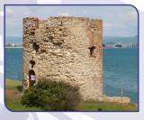
It is located on the north coast of the peninsula next to the remains of the Basilica of Virgin Mary Eleusis. The huge body of the mill is a regular cylinder with massive walls, built of crushed stone, excavated on site. Through the arched door, which has a stone block frame, you enter the ground floor, which served as a store-room. A massive staircase of oak logs leads to the second floor. The working room of
